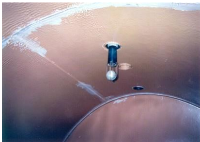
Flow Restriction (Ball Float Valve)*
