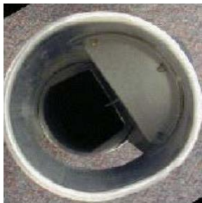
Automatic Shutoff Device (Flapper Valve)
